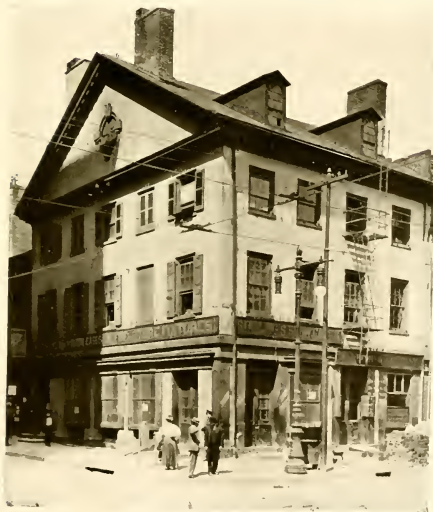
HOUSE OF REV. WILLIAM SMITH, D.D., FIRST PROVOST OF THE UNIVERSITY OF PENNSYLVANIA, NORTH- EAST CORNER OF FOURTH AND ARCH STREETS
